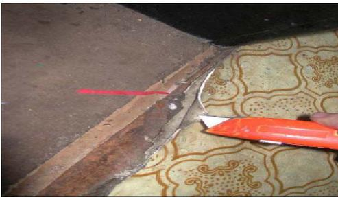
Figure 1 - Asbestos backed vinyl sheet flooring
