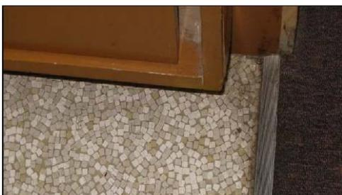
Figure 2 – Terrazzo type asbestos backed vinyl sheet flooring.
