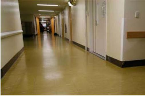
Figure 3 – Asbestos vinyl tiles © Worksafe Victoria
